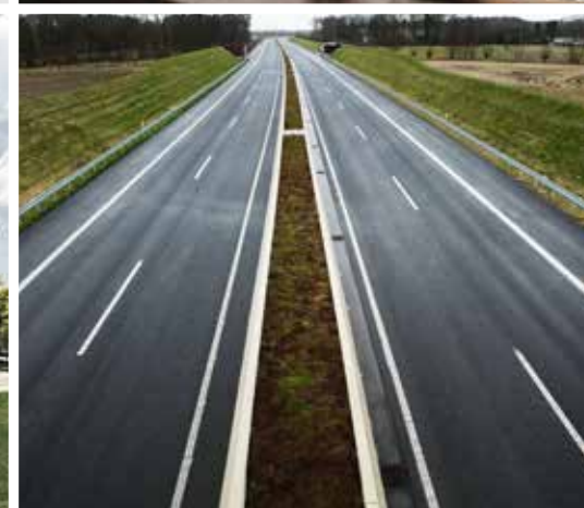
ACCESS TO HWY 401
